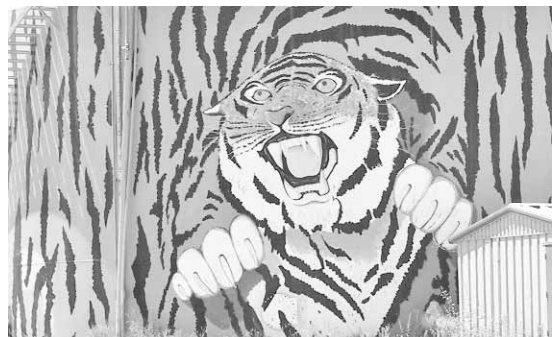
The Tiger Tank is one of several storage tanks for water in the Village of Los Lunas.
